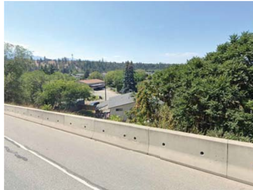
2. VIEW FROM SPRINGFIELD ROAD FACING THE SITE
