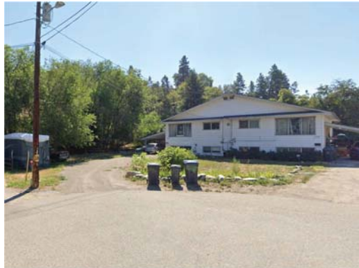
1. VIEW FROM MONTEREY CT FACING THE SITE
